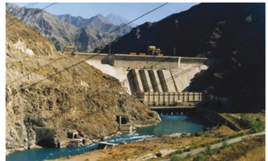
Fig. 2 Construction of Kambaratinskaya HPP-2.
